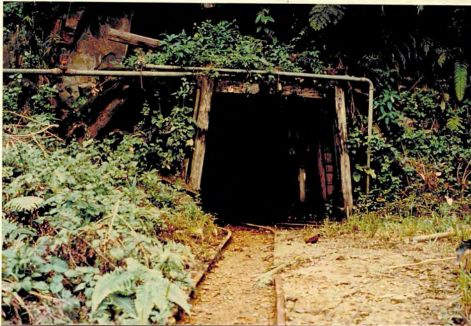
Plate 12. The entrance to tunnel T.580, which is completely in monzodiorite.
